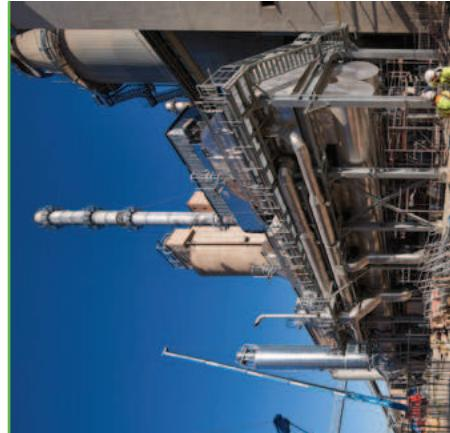
In 2019, OPTERRA, part of our Europe Materials Division in Germany, installed new exhaust gas purification system at its Karsdorf cement plant. The new filter technology, which includes a state-of-the-art AUTONOX® Low Dust System installed on the existing kilns, enables the cement plant to comply with the new limits for dust, ammonia and nitrogen oxide emissions introduced in Germany.
